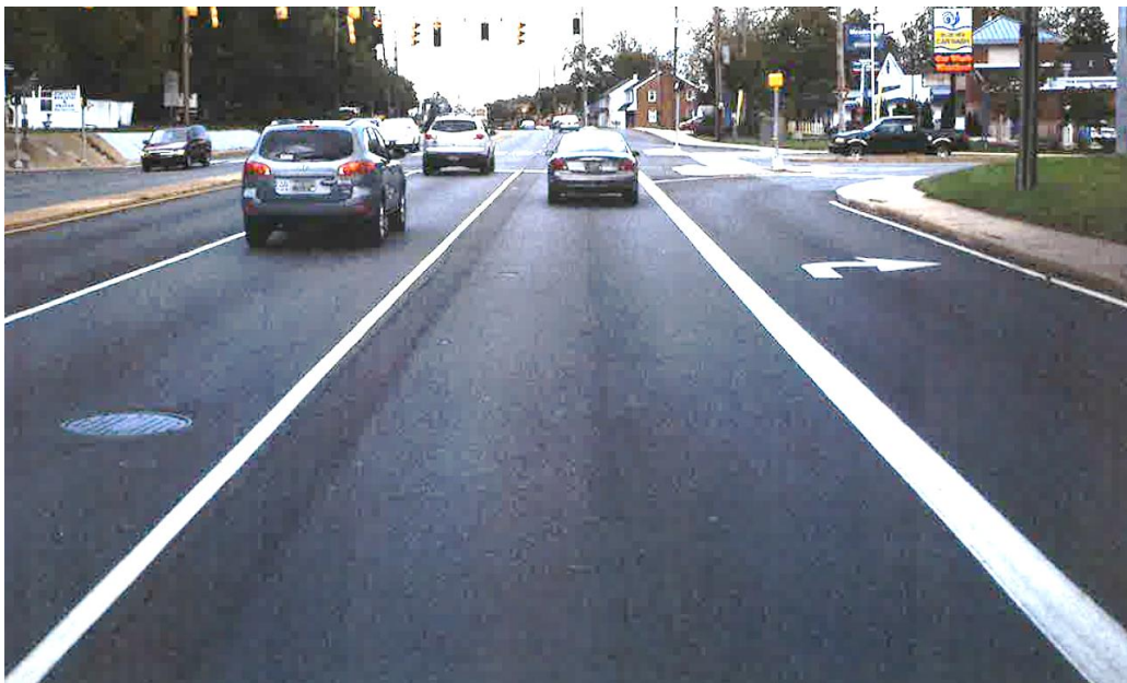
Figure 7: Example of a primary arterial composite pavement in excellent condition with OPC 90.5
