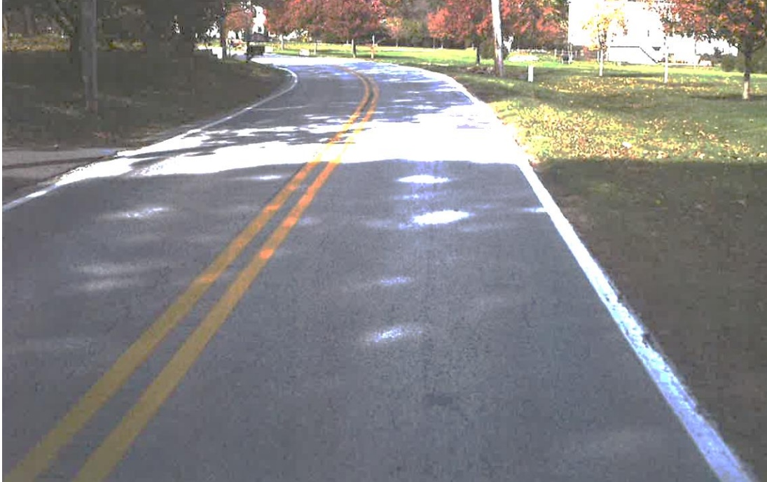
Figure 8: Example of major collector pavement in good condition with OPC 72.0
